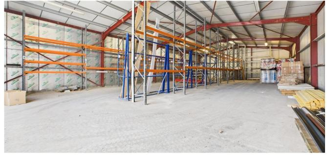
The subjects comprise of a detached industrial unit of steel portal frame construction with a pitched roof over clad with insulated profile metal sheeting.
