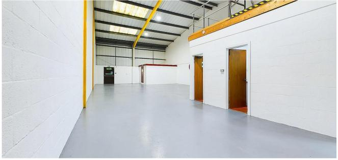
The unit is of a steel portal frame construction with brick dado walls and clad thereafter with PVC coated pressed steel cladding. The roof over is similarly clad and incorporates a number of roof lights.
