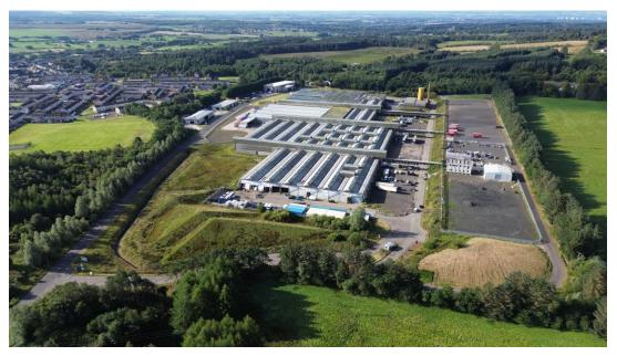
The subjects comprise a substantial warehouse and distribution hub of steel portal frame construction with profiled aluminum cladding and pitched roof. The property benefits from various pedestrian entrances along with a number of vehicular roller shutter doors.
