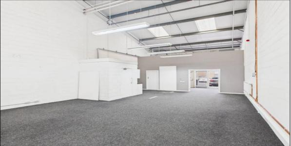
The subjects comprise a variety of mid and end terraced office/industrial units within a single storey multi-let block. The building is constructed of steel frame with block infill walls, surmounted by a pitched profile metal sheet covering, incorporating translucent panels.
