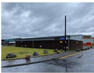
The subjects comprise a detached building of steel portal frame construction part infilled with concrete block clad externally with profile metal sheeting and harling and with mono pitched profile metal sheet roof over.
