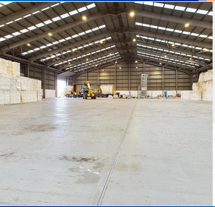
The subjects are of a steel portal frame construction with concrete block walls to dado heigh and profile metal sheeting thereafter. The roof over is pitched and with profile metal sheeting and incorporates translucent roof panels.
