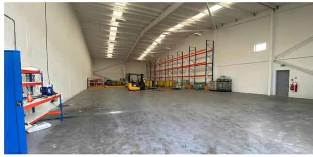
The subjects comprise of an end terraced industrial unit and is of a steel portal frame construction with a pitched roof over incorporating translucent roof panels along with a single storey office of blockwork constriction with a flat roof over. The space is laid out to provide warehouse and office accommodation.
