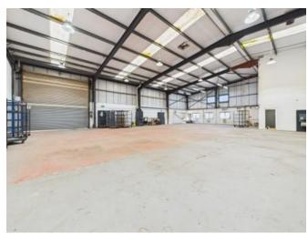
The property comprises a semi-detached industrial building of steel portal frame construction incorporating two storey offices at the front elevation. Externally the building has been clad with profile metal sheeting within the workshop area and brick to the office area. The roof over is pitched with a profile metal roof over.
